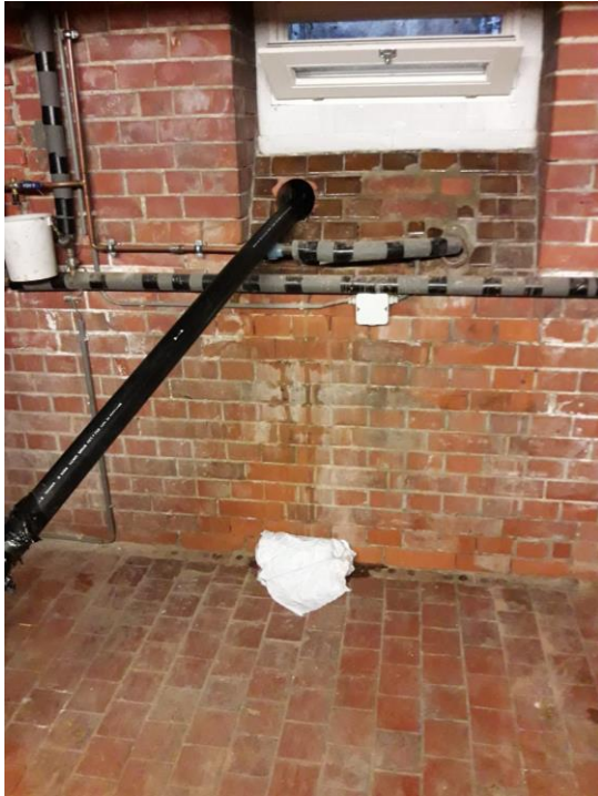
Foto: Holland Drilling
