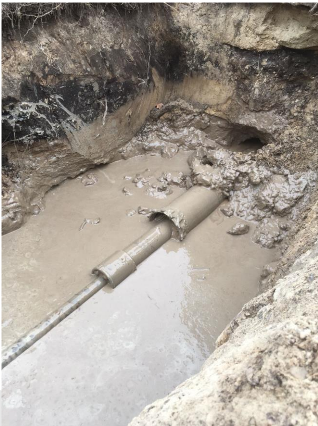
Foto: Holland Drilling
