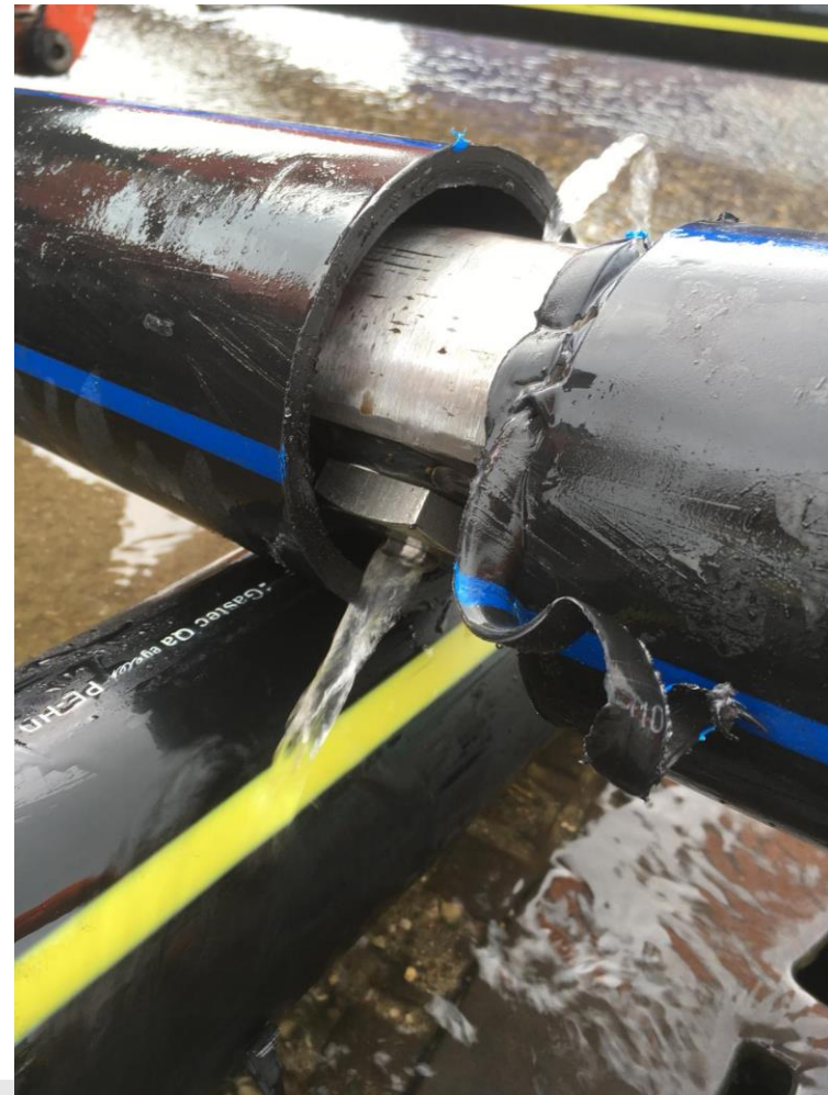
Foto: Holland Drilling
