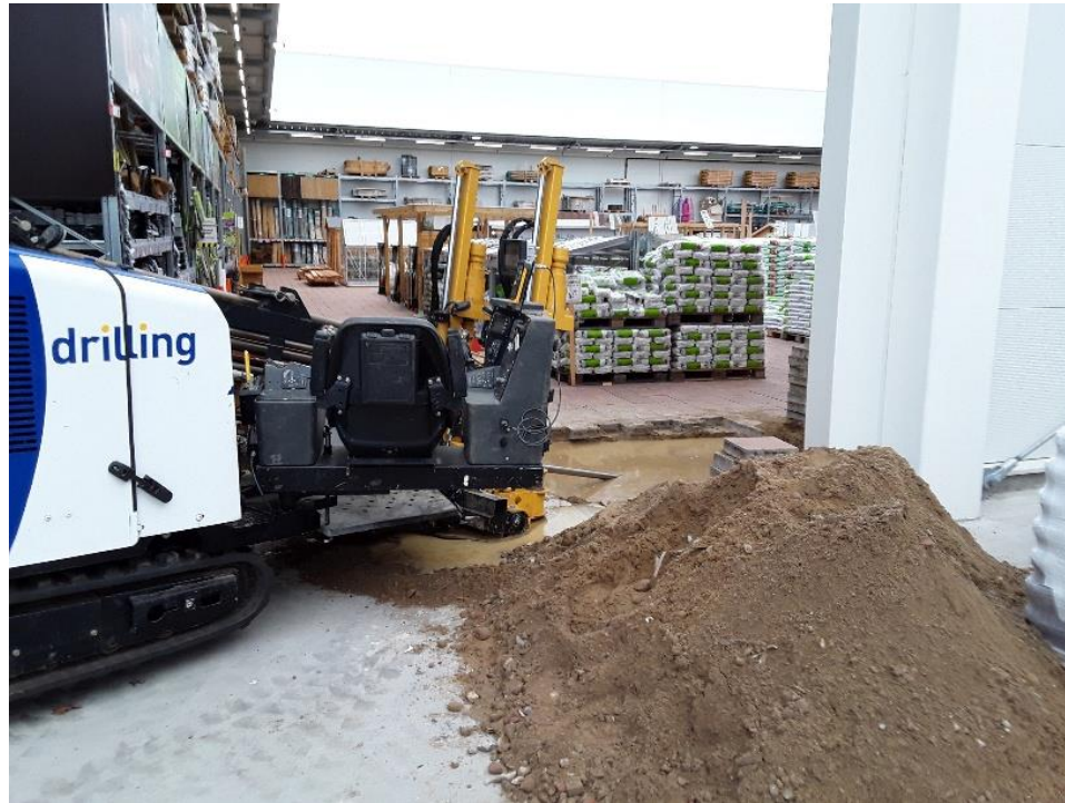
Foto: Holland Drilling
